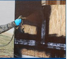
Seals sheathing joints, preventing air and water infiltration & damage.
