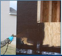
Uniformly coats and protects sheathing from liquid moisture penetration, but allows vapor to escape.
